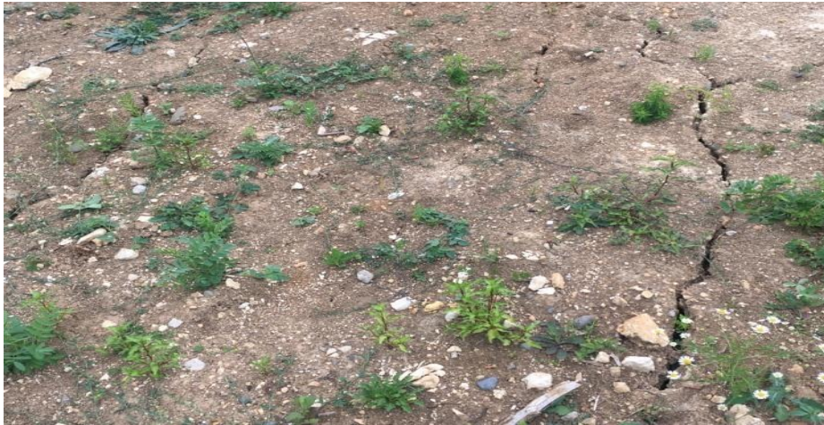
Cracks on the ground surface at the spoil disposal area (landslide hazard)
